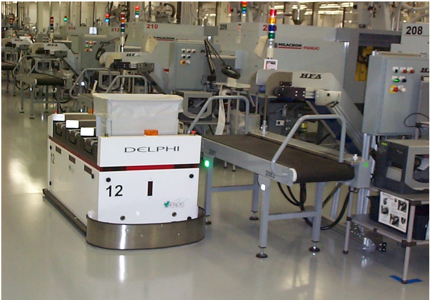
2250 “Z” Style Conveyor Feeding a Tote-Loading / Unloading Station
