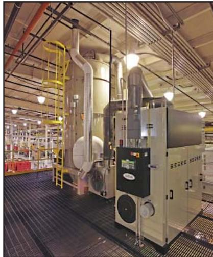
**Desiccant-wheel dryers, such as this Conair W5000, are being used more and more as a cost-saving solution for large central drying systems.**
